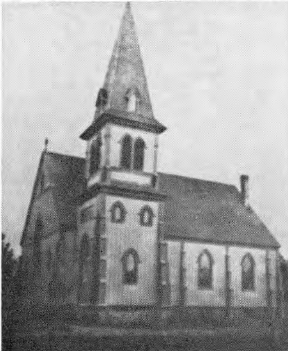
Hillsdale Methodist Church — 1900
