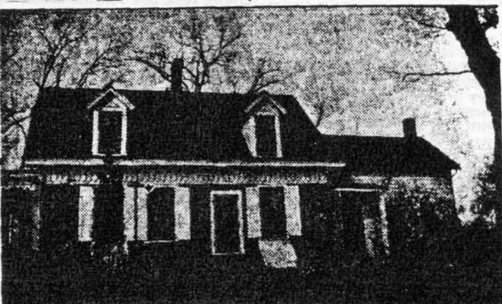
The old Samuel G. Demarest Home as viewed from the West is one of the more perfect examples of the colonial type architecture which predominated in Hillsdale at the turn of the century. It is reputed to have been built in 1815. The lower home, now known as the Armstrong House on Ell Road is a claimant for honors as the oldest home in the Borough. It was built long before 1800.
