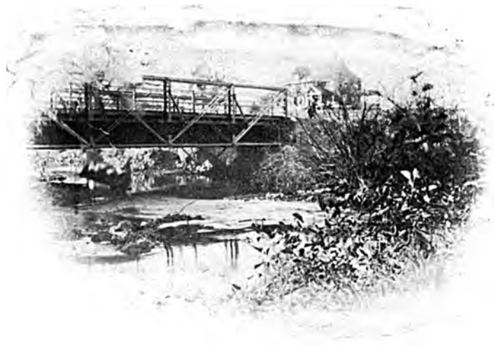
Bridge Crossing the Hackensack at River Vale. .
