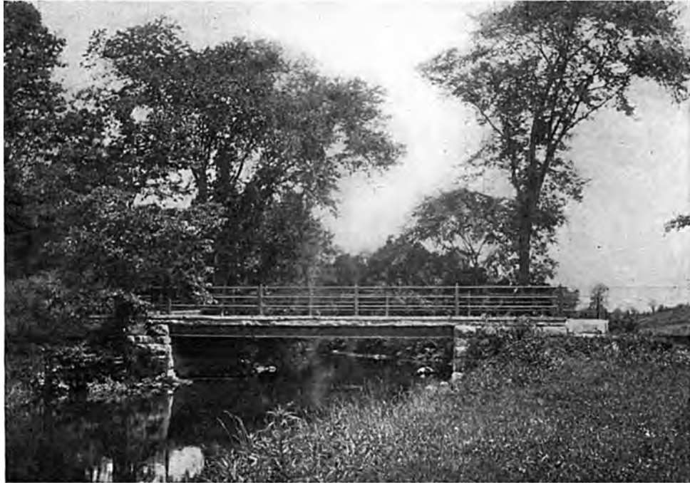
Hillsdale Avenue Bridge.
