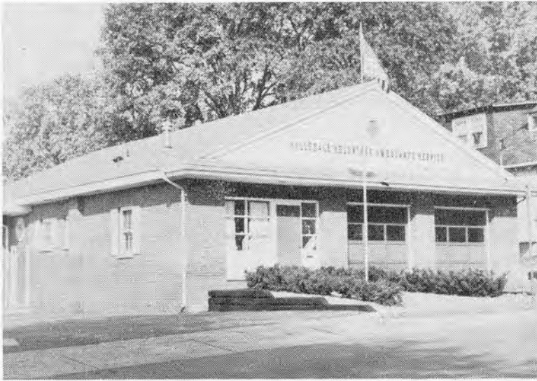
Hillsdale Volunteer Ambulance Bldg.
