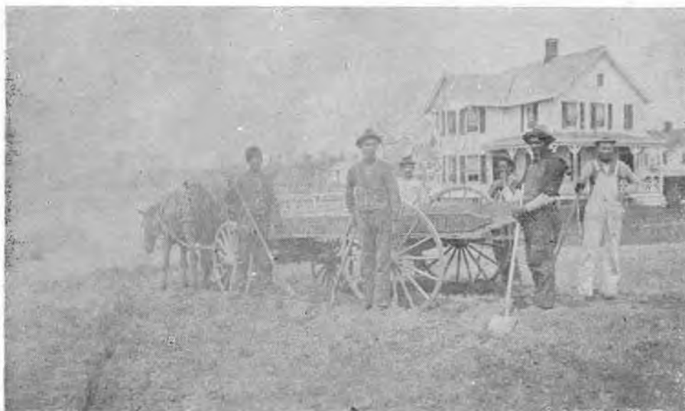
Working on the Roads of Hillsdale — 1899
